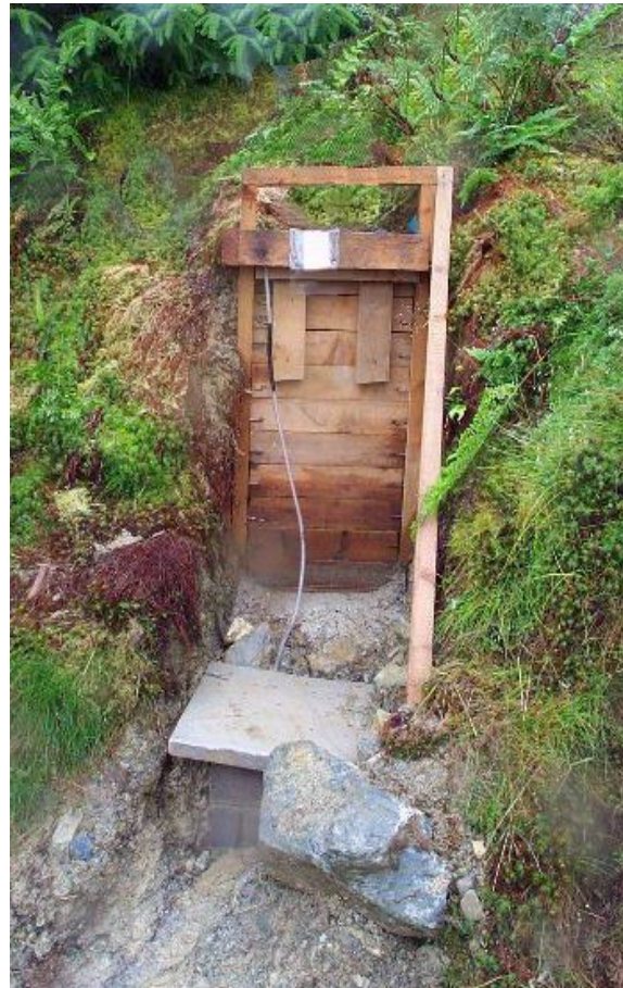
Figure 3.41(b) Site after installation of water flow recorders and data loggers, Pared yr Ychain
