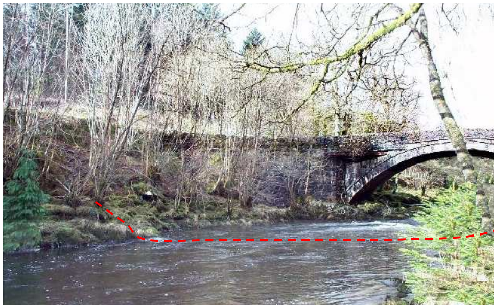
Figure 3.20(b) (above) Line of cross section surveyed at Pont Dolgefeiliau, Afon Eden
